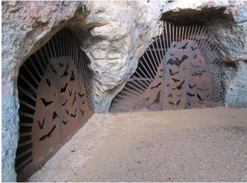
Figure 17. Closure of the Waterkuil, one of the largest quarries of Henisdael.
