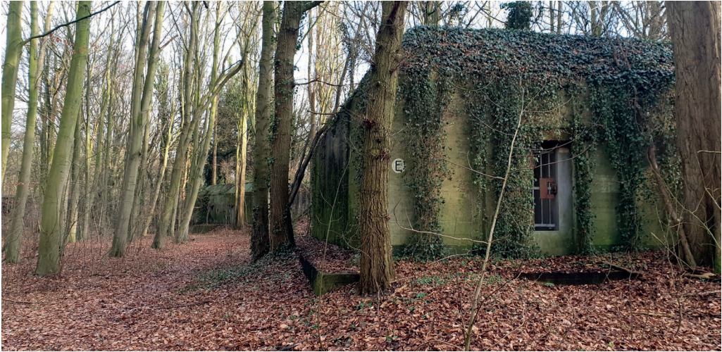
Figure 4. Above-ground bunker Staelduinse Bos, Hoek van Holland. Photo: Kees Mostert.
