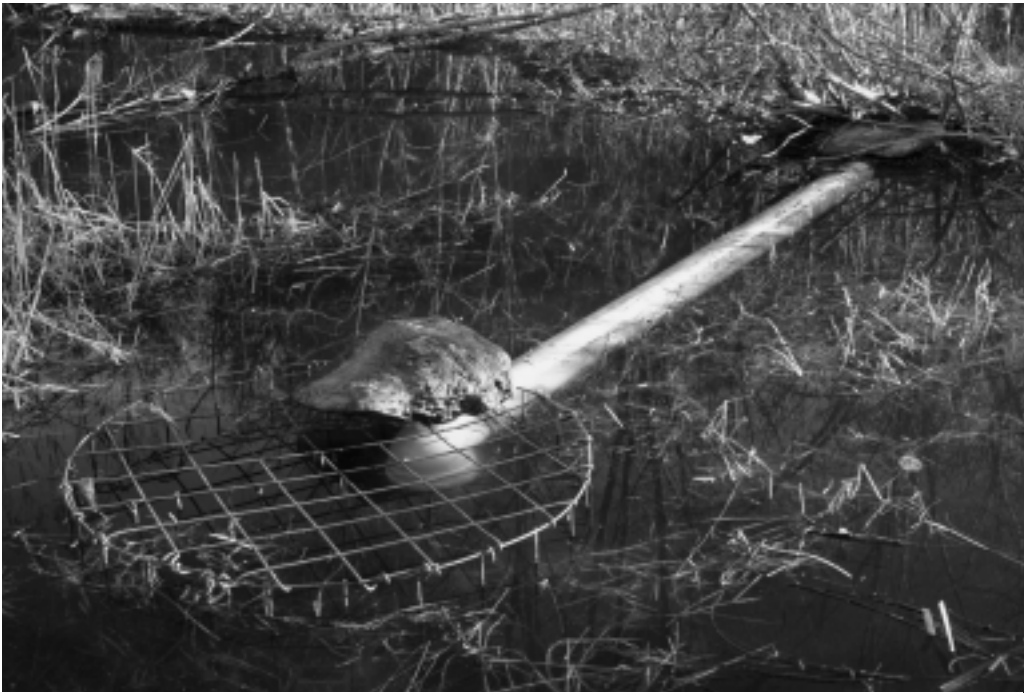
Photo 1. Castor Master™ pipe systems use a Round Fence™ (RF) for a filter. Many types and sizes of pipes can be used; this one is of polyvinylchloride and measures 0.2 x 4 m. Because the pipe is placed level it has a silencing elbow to prevent the sound of running water from escaping and attracting beavers. This RF is small (diameter: 1.2 m) and lightweight so it has a rock on top of it to help counter liquid-displacement forces acting on the pipe. The pipe is also weighted down where it ends in the dam and covered with branches so beavers cannot access it. This is a relatively small system to match a small stream. Photograph: Skip Lisle.
