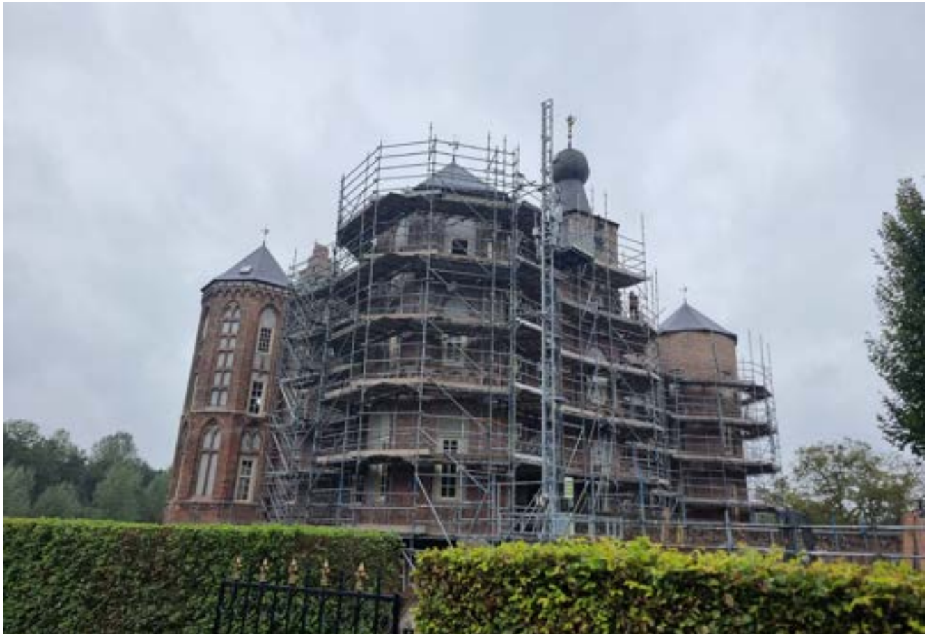
Foto 9 | Kasteel Croy in de steigers.
