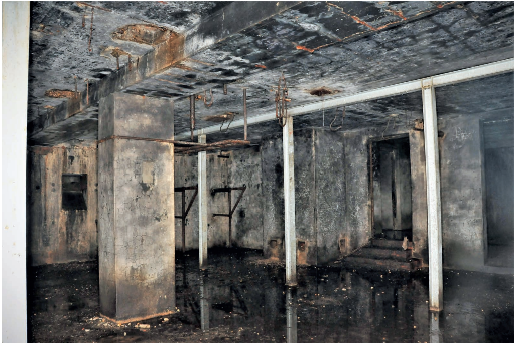
Figure 2. Interior of the largest cellar (KHK1). Photo: Ruud Kaal.
