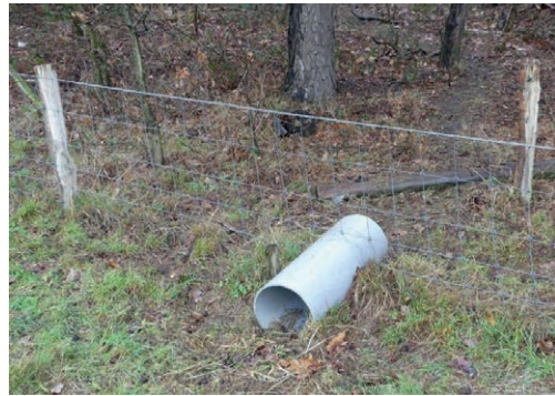
Figure 3. PVC tube, 0.3 m diameter, across a fence enabling badgers to visit their feeding grounds. Photo: Hans Vink.
